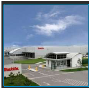
Name: MAKITA FACTORY Country: Branesti, Romania
