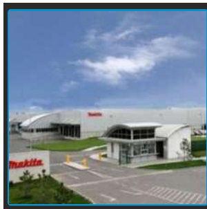
Name: MAKITA FACTORY Country: Branesti, Romania
