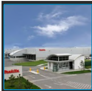
Name: MAKITA FACTORY Country: Branesti, Romania
