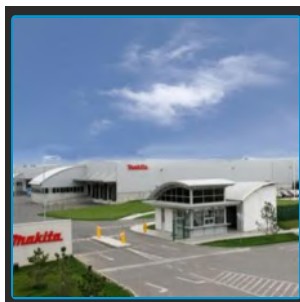
Name: MAKITA FACTORY Country: Branesti, Romania
